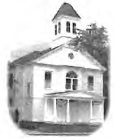
Ye Olde Court House - Masonic Hall
